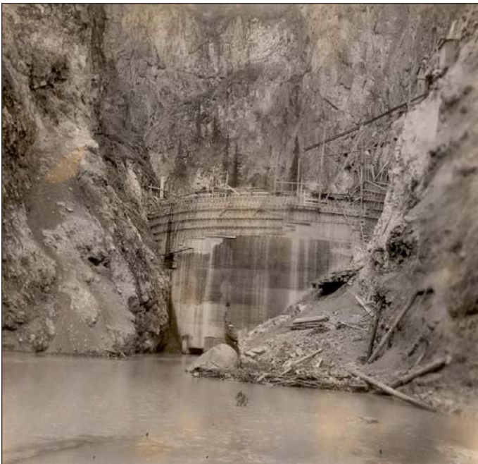
Figure 12. Upstream face of diversion dam under construction.
