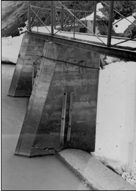
Figure 13. Catwalk installed on diversion dam in 1933 at request of FPC. Courtesy of National Archives, AK Region, APA Box 42.
