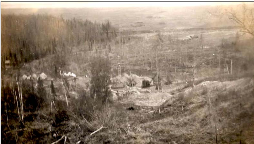
Figure 10. View of construction camp at powerhouse site – note tents, center, left (circa 1928).
