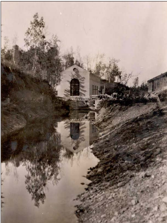
Figure 19. Tailrace extending from rear of powerhouse.
