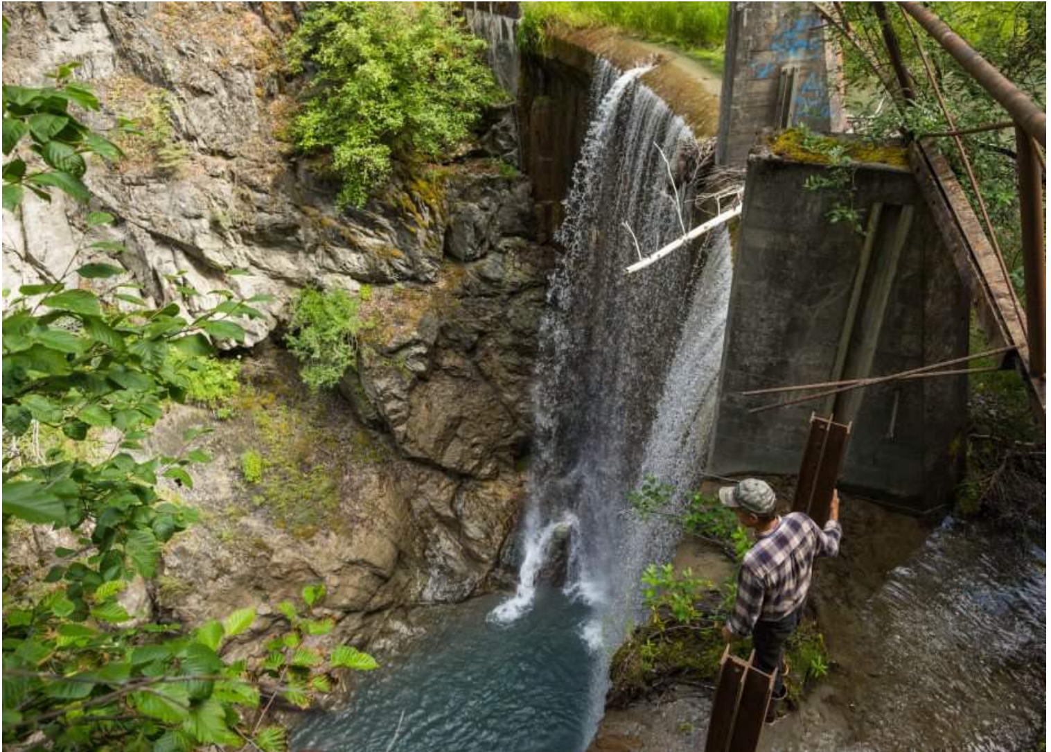
Rick Sinnott peers over the lower Eklutna River dam on Thursday, July 23, 2015. The obsolete 61-foot high dam, built in 1929, may soon be dismantled, allowing salmon to return to the river. Loren Holmes / ADN
